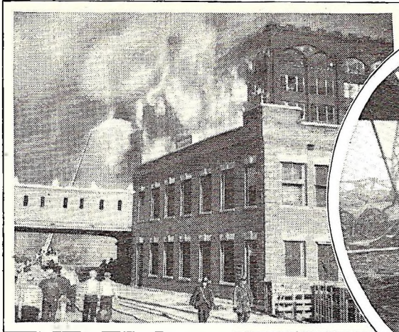
The nine story Exchange Building shown here was the tallest structure destroyed in Chicago's recent fire.
